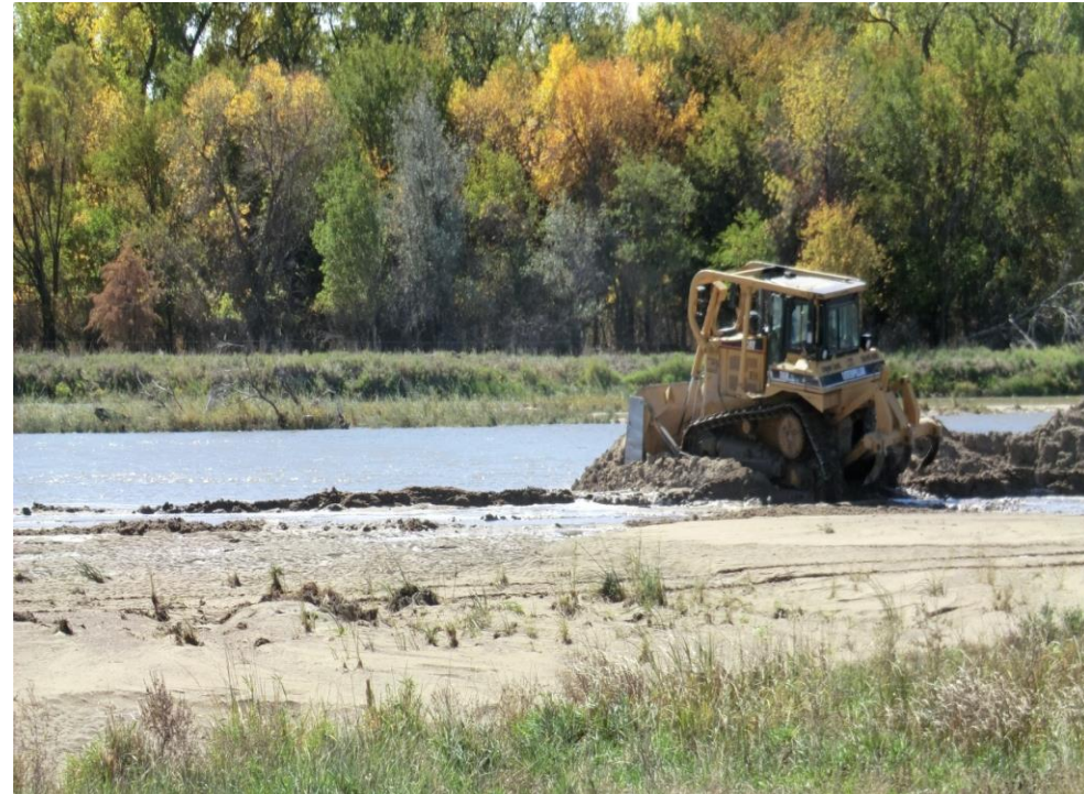
Mechanical Creation & Maintenance (MCM) “Clear/Level/Plow”
